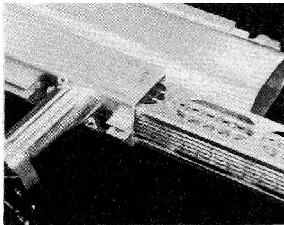
Fig. 11 Al-distributed sputter ion pump is housed in the bending magnet vacuum chamber. Left side is the pumping port.
