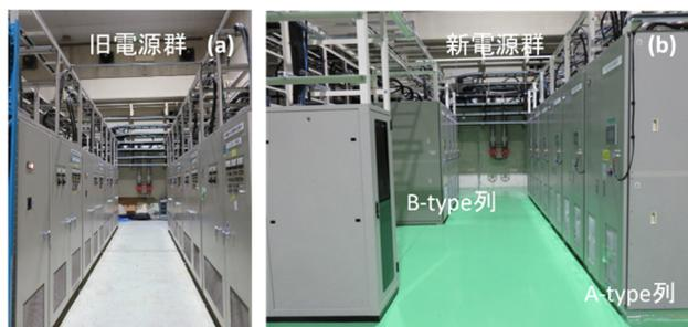
Figure 4: Old and new power supplies for quadrupole and sextupole magnet.
