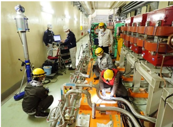
Figure 3: Marking the center of the electromagnet and the tapped hole position
