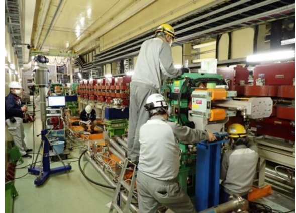
Figure 4: Alignment of quadrupole magnets
