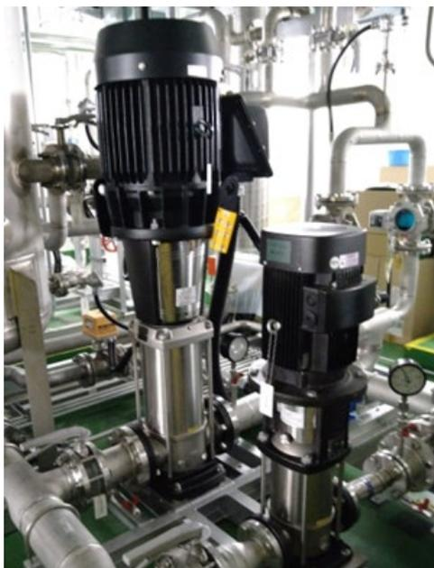
Figure 6: A large water pump for normal operation and small one for standby operation in a night.
