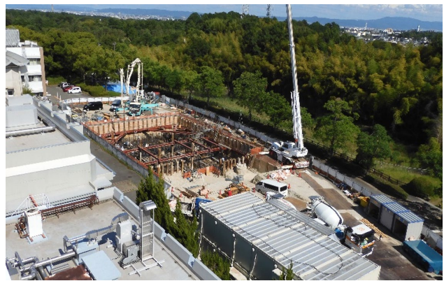
Figure 3: Construction of new building for 211At distribution.
