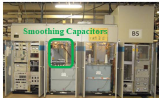
Figure 1: The modulator of KEK electron/positron linac.
