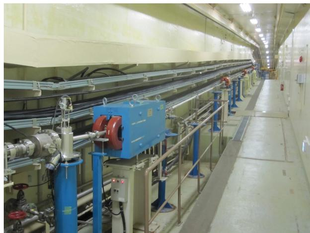
Figure 1: Photo of the PF-BT. The PF-BT is a 2.5 GeV beam transport line with a total length of about 170 m and connects the end of the LINAC located underground to the injection point of the PF-ring located at ground level.
