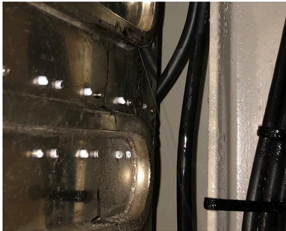
Figure 10: Leakage of cooling water of the cooling plate of transistors in the power supply for the sextupole magnet.
