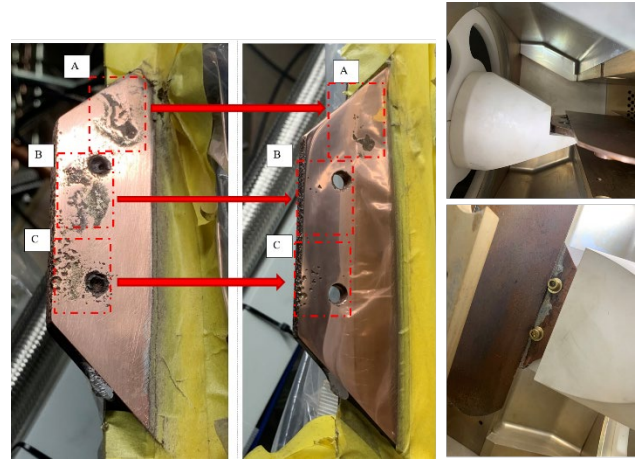
Figure 5: On-site repair for the port-1 (2022/June).
