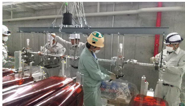
Figure 5: Installation of vacuum chamber.
