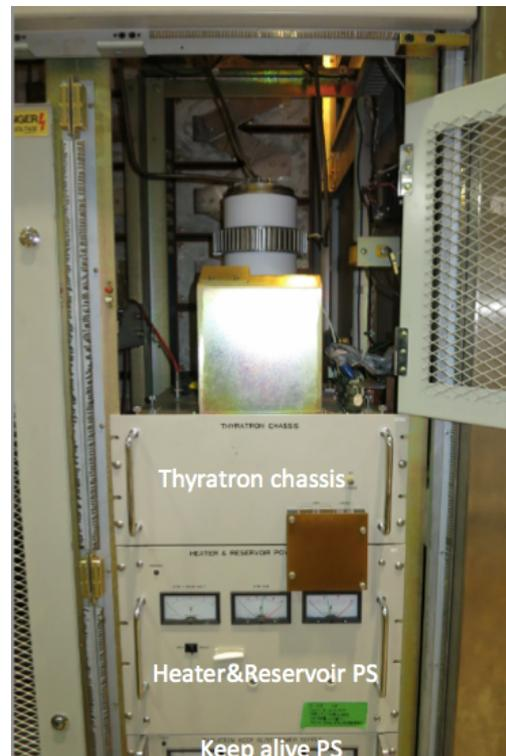
Figure 1: Thyatron switch tube installed in modulator.
