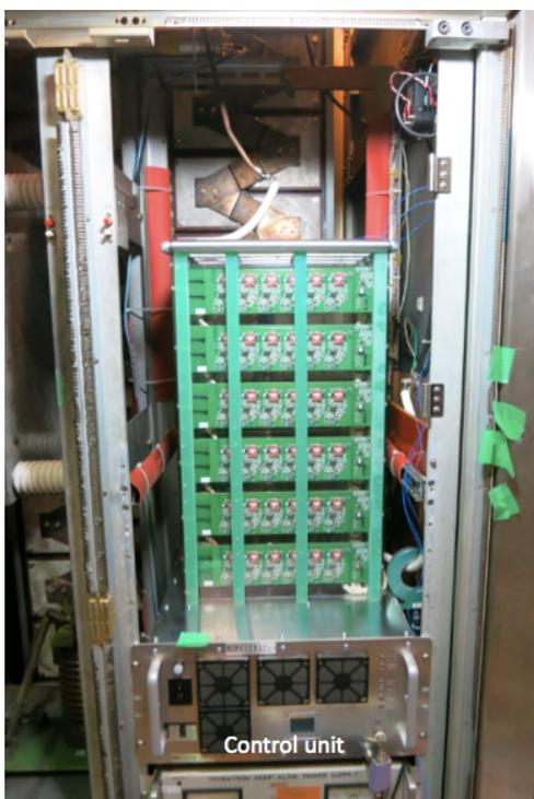
Figure 2: Solid-state thyatron replacement switch installed in modulator.
