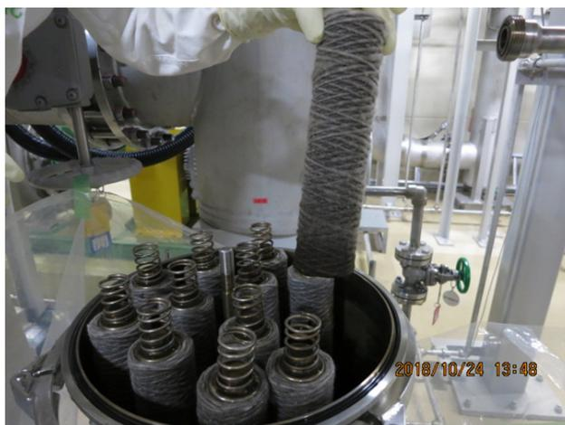
Figure 5: Replace a filter of RI4 water cooling system in J-PARC Linac.
