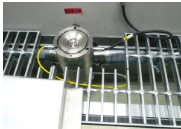
Figure 6: HLS in the tunnel pit.
