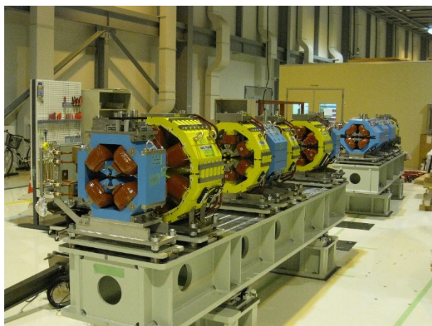
Figure 4: B-girder and C-girder installed at the test half-cell in the SPring-8 experimental hall.
