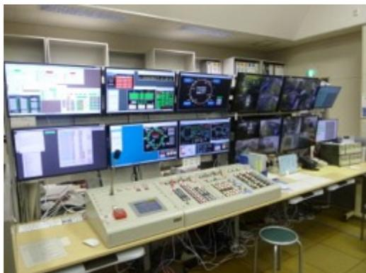
Figure 5: The safety system console.
