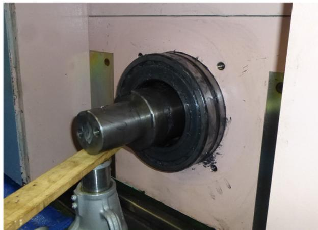
Figure 3: Replacement of a bearing used in a shielding door.
