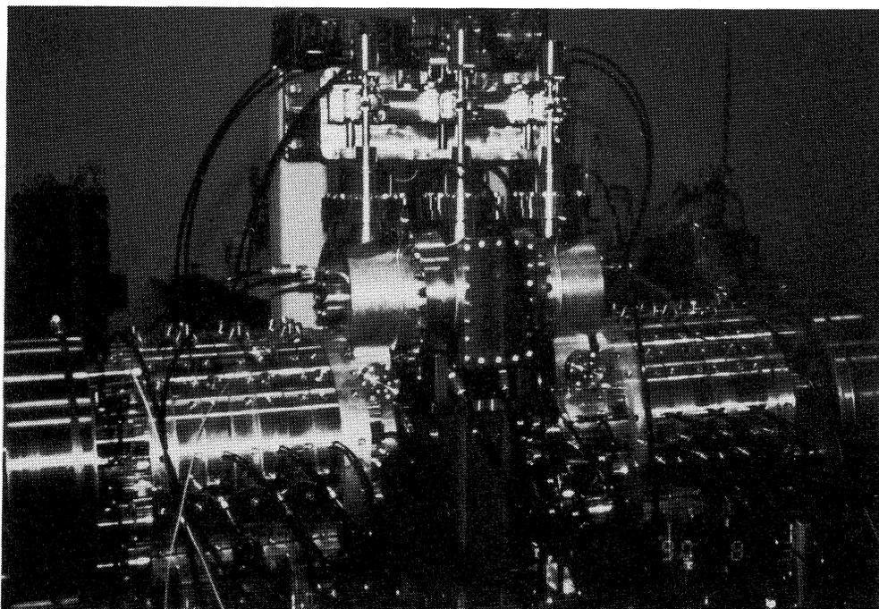
PHOTO Assembled Bridge Coupler-Accelerating Tank System
