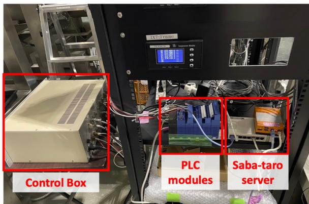
Figure 3: Real implementation of a PLC controller, a micro-server, and a control box in KAGRA.
