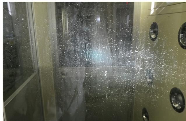
Figure 1: Window of air shower between STF class 1000 and class 10 clean room.
