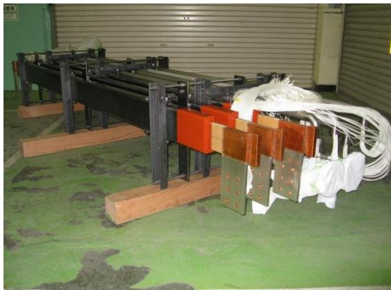
Figure 9: P6 utility duct (signal cable ducts, electric power bus ducts, water pipes, a vacuum pipe)
