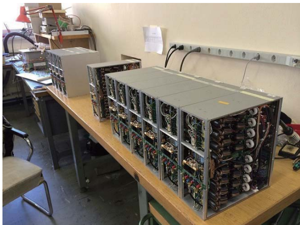
Figure 6: Solid State Amplifiers for CERN PS Booster.
