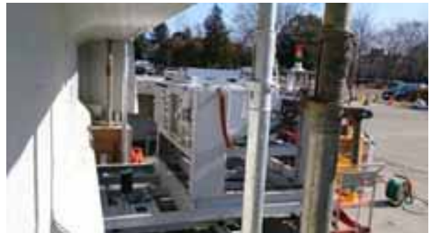
Figure 5: On-site non-destructive measurement of bridge structure with 3.95 MeV X-band Linac.
