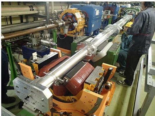
Figure 5: Aluminum-alloy beam pipe installed into the quadrupole and sextupole magnets in arc section.
