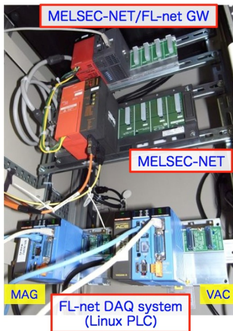
Figure 3: Data acquisition system for the vacuum and magnet protection interlock system at slave 25 rack.
