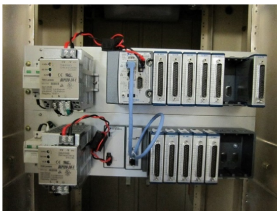
Figure 5: CompactRIO under installation. The light blue cable is used in order to interconnect the EtherCAT slave chassis (down) to the EtherCAT master controller (up).
