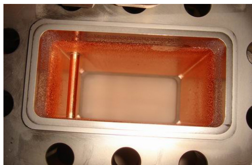
Figure 2: Status of a water leak in a wave guide of 5th accelerator tube.
