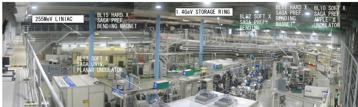
Figure 1: Present status of the experimental hall of SAGA-LS.
