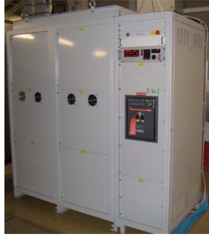
J-PARC (Tokai) SCRs technology (12/24 pulses) up to 20 kA Efficiency at P_{max} >90%
