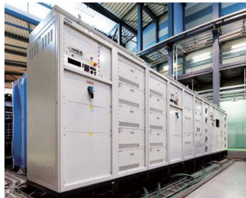
ALBA synchrotron (Barcelona – SPAIN) Ramped PSU 1000 V/750 A
