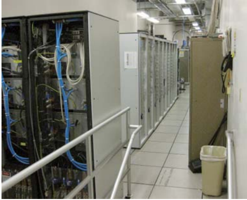
MGH Boston (USA) PSU for Dipoles, quadrupoles Proton therapy, 2 or 4 quadrants, secondary Switch mode, 200 V/200 A
